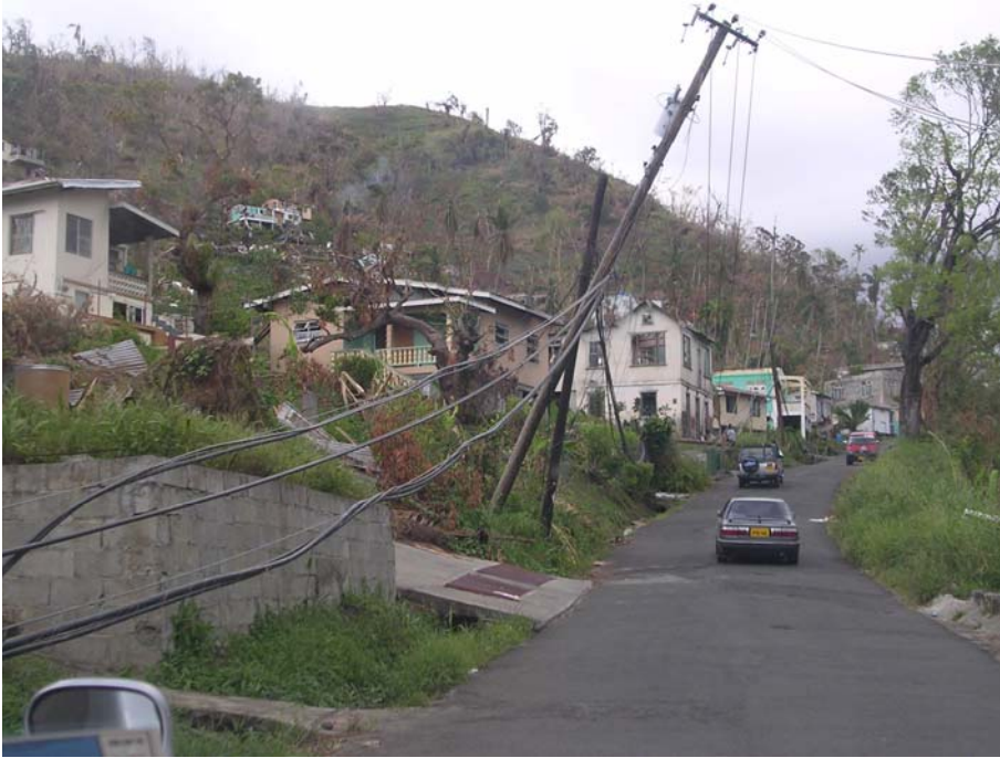
Photo 7 Downed Poles Carrying Communication Cables
