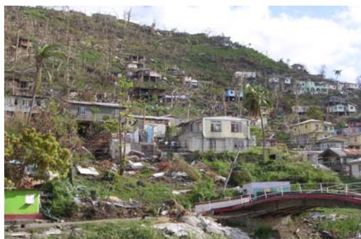
Photo 1 Damaged Housing in St. Georges
