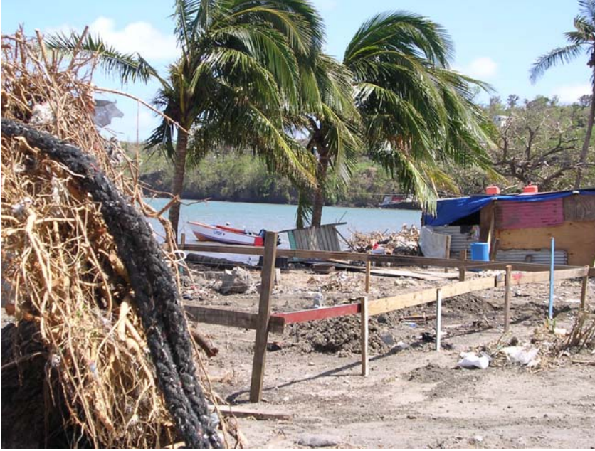
Photo 11 Reconstruction of housing at Soubise/Marquis
