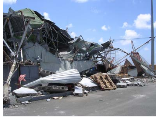
Photo 14 Damaged Geest Warehouse
