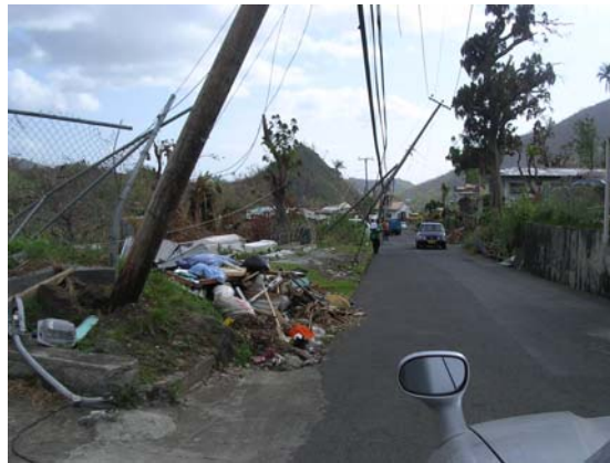
Photo 4 Typical Damage to Electric Poles
