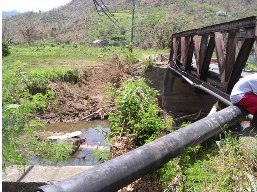
Photo 6 Damaged Water Supply Infrastructure at Beausejour
