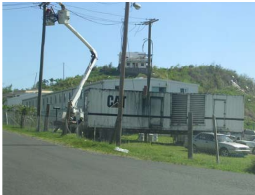
Photo 5 1.5 MW Unit in Lance Aux Epines
