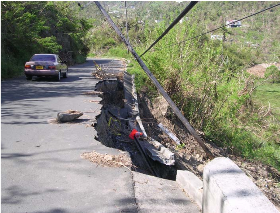
Photo 9 Erosion of Roadway at Westerhaul
